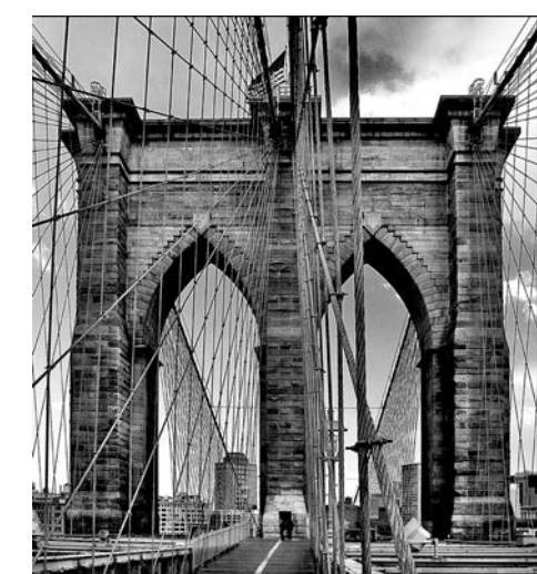
Work by H. Scott Cushing
