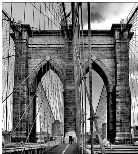
Work by H. Scott Cushing
